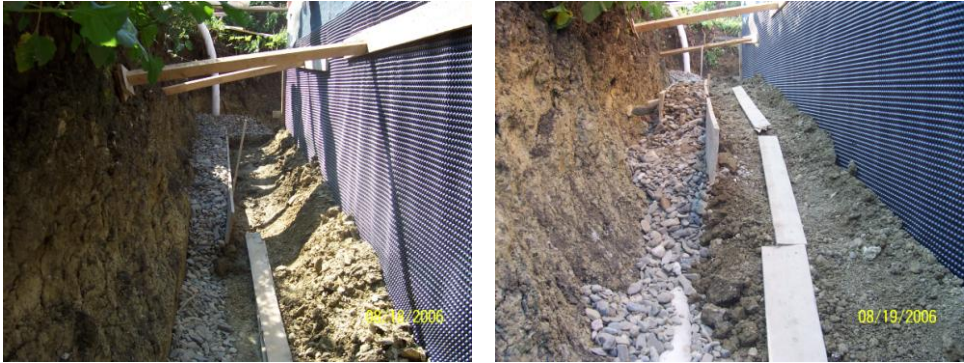
Fig. 4 – Placing the filter material on the drainage tube
