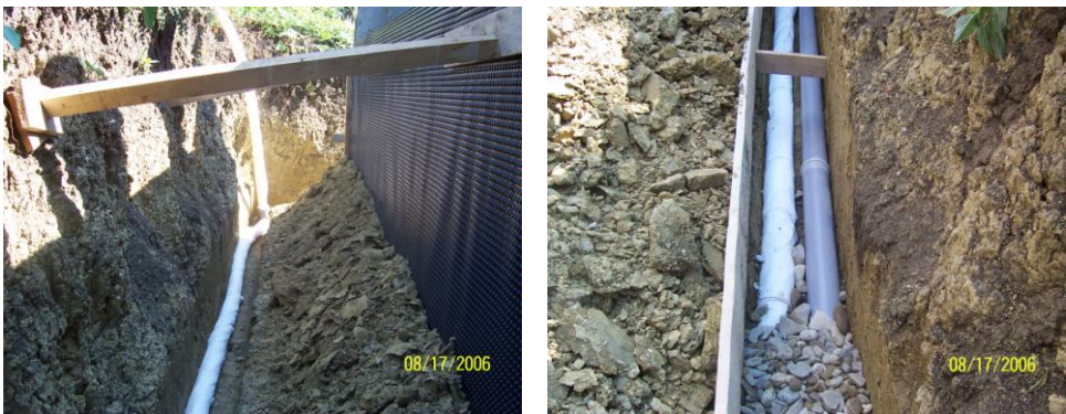
Fig. 3 – Laying the drainage tube wrapped with geotextile
