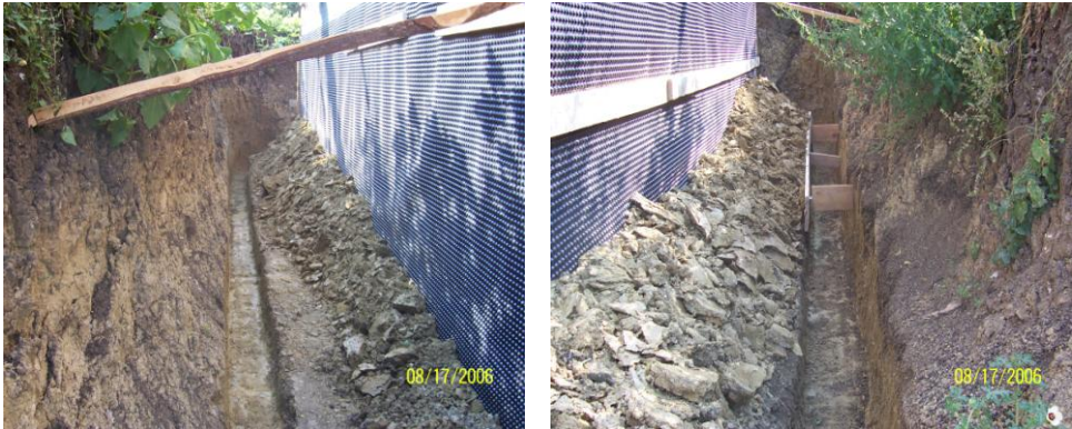
Fig. 2 – Channel execution for laying the drain
