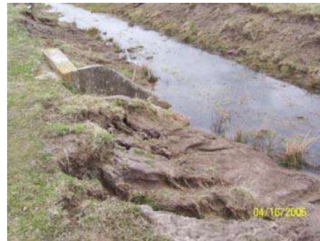
Photo 5 – Slope erosion and channel bottom silting
