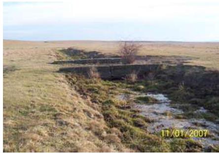
Photo 2- Channel section and silted footbridge
