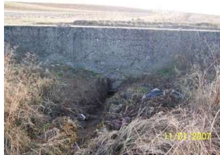
Photo 2- Channel section and silted footbridge
