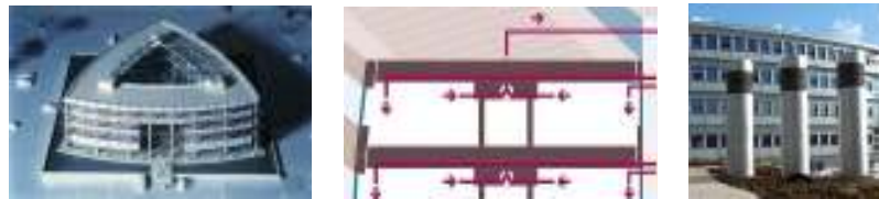
Fig. 3 – Overview of the EnerGon building exterior (left), natural ventilation circuit diagram of the last level (middle), air vents absorption system for underground wells (right), (Faigle B.,2005), (Lindemann, 2007)
