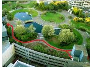
Fig. 3 - Intensive roof garden ( www.naturalpatriot.org )
