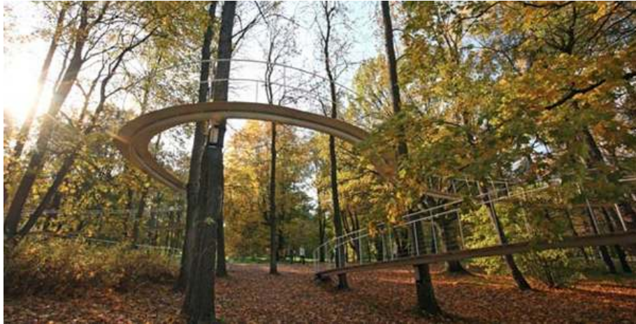
Fig. 2 - The installation called A path in the forest is a suspended bridge, sustained exclusively from the trees trunks. An event is created, a surprise in the landscape path. The intervention is reversible and does not aggressively intervene in the natural habitat of the forest. Tallinn, Estonia, 2011, autor: Tetsuo Kondo, Photo credits: © thecoolhunter.net
