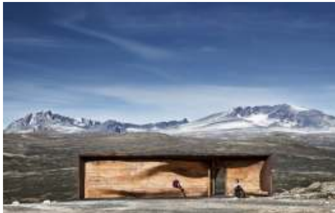
Fig. 1 - Norwegian Wild Reindeer Centre Pavilion, Hjerkind, landscape architects Snøhetta Oslo AS the inner wooden shell shaped by means of computer aided design and advanced processing technologies
