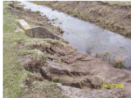
Photo 5 – Slope erosion and channel bottom silting
