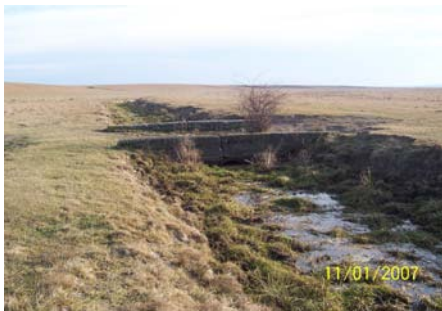
Photo 2- Channel section and silted footbridge
