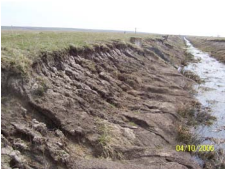
Photo 5 – Slope erosion and channel bottom silting
