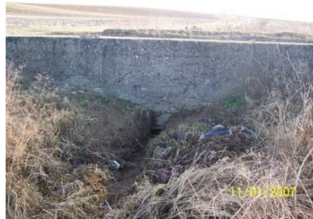
Photo 2- Channel section and silted footbridge
