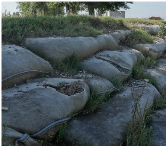
Figure 12 Degradation of the geo-bags located at the top of the coastal defence by anthropogenic actions (photo author, 2022)
