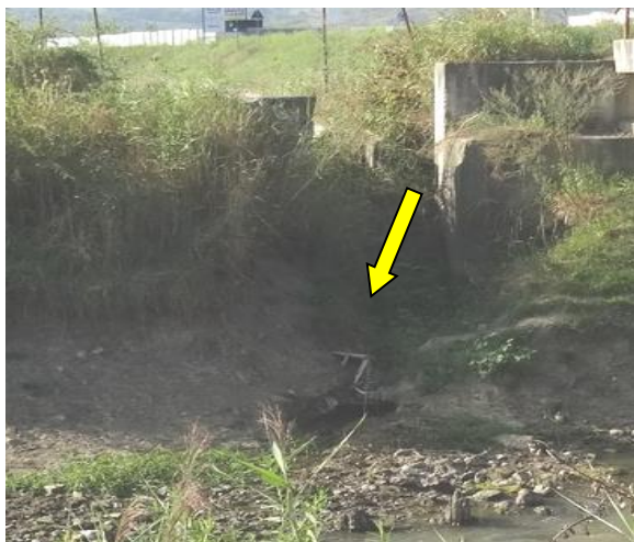
Figure 10 Intense phenomenon of erosion on the right bank of the Bahlui River bed at the outlet of perimeter channel 2 (Luca M., 2019)
