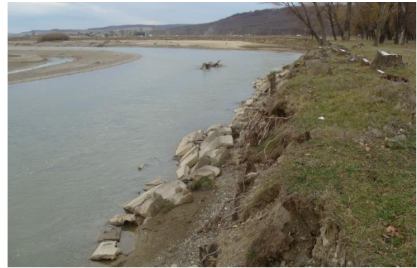
Figure 5 The total degradation of the defences on the left bank of the Moldova River, year 2012 (Luca M., 2012)
