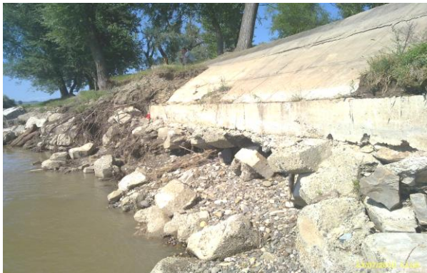
Figure 4 The structural state of the shore defence made of concrete slabs in 2008 (Luca M., 2012)
