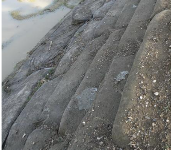
Figure 11 Degradation of geo-bags in contact with water in the flood of 2018 (photo author, 2018)
