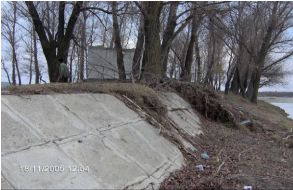
Figure 3 The structural state of the left bank defence on the Moldova River in 2005 (Luca M., 2006)
