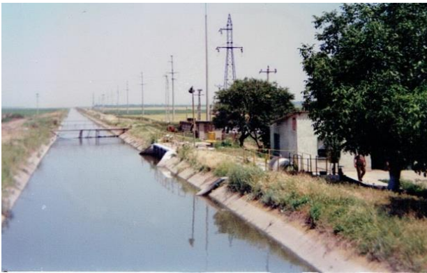
Figure 3 Irrigation canal made in semi-embankment with water intakes for pumping and pressurization stations, SPP (Ghelase I., 2000)
