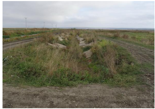
Figure 9 - General view of the CA3 canal and a modified bridge at the intersection with an exploitation road (Luca M., 2020)
