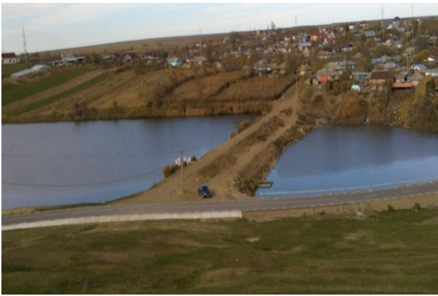
Figure 2 Overview of the Podișu earthdam (photo: Agapie I., 2019)
