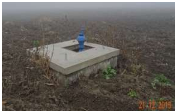
Figure 8 Rehabilitation of the ventilation chimney on the main pipe CP1 in "Berezeni Plot 16" (Luca, 2015)
