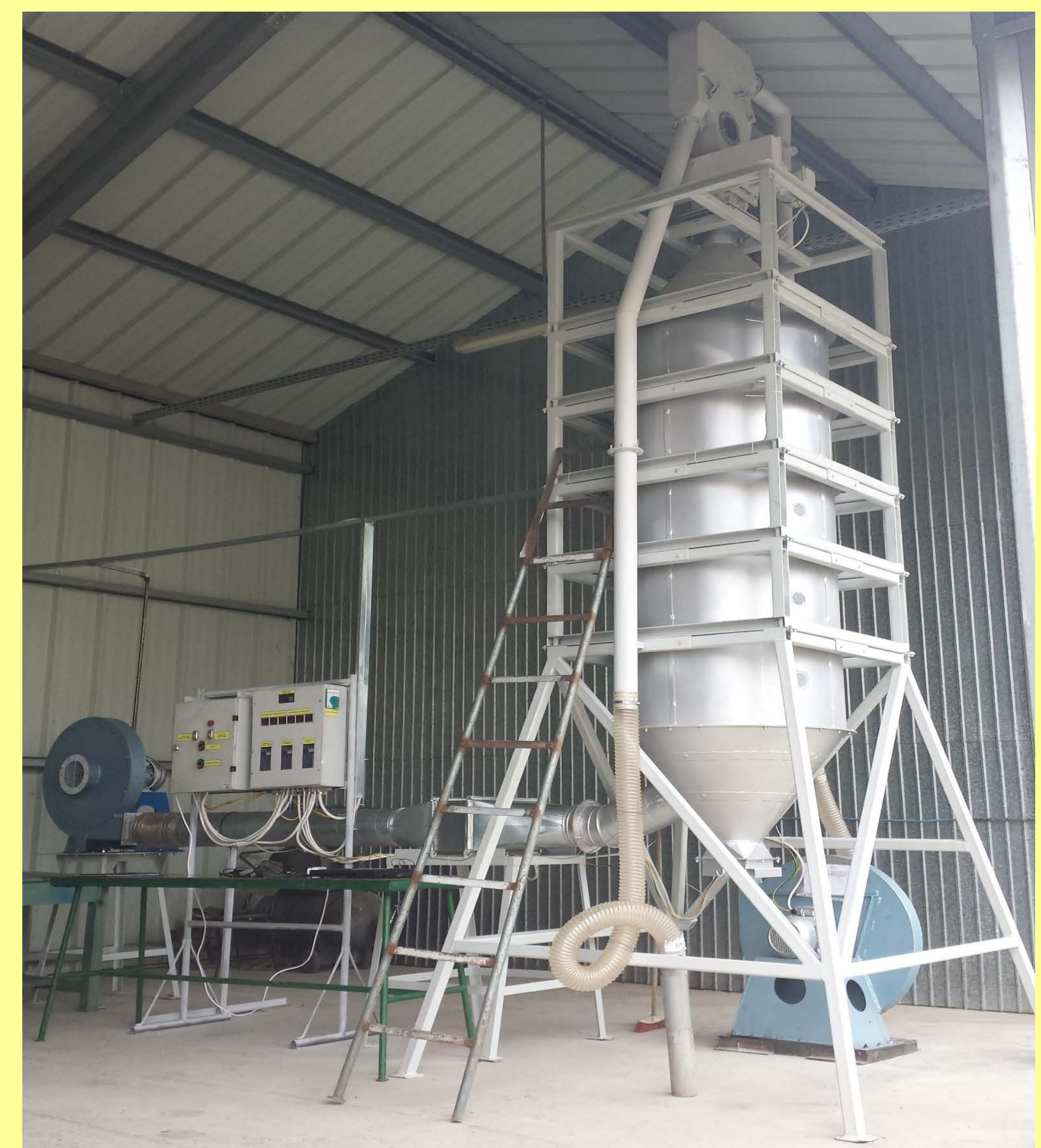
Innovative model of vertical dryer with heat recovery
