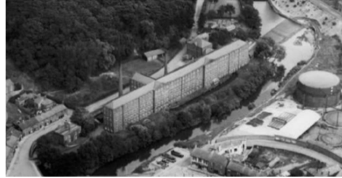
Fig. 2 - Old Mill, EastCheshire, aerial view, half of the 18th century
