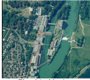
Fig. 14 - Menier chocolate factory, Noisiel-sur-Marne after the conversion
