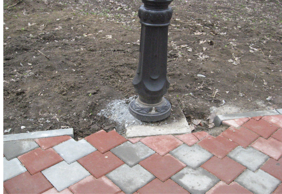
Fig. 3 - The edge is interrupted by wrong position of public lighting columns (photo D. Dascalu)
