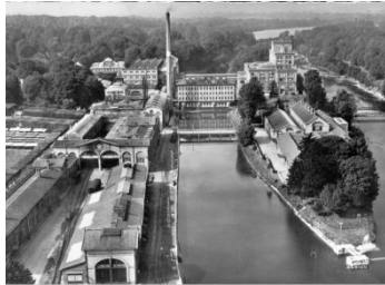
Fig. 12 - Menier chocolate factory, Noisiel-sur-Marne. Archive image before the conversion
