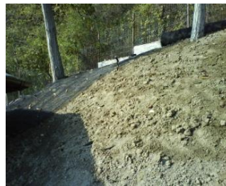
Fig. 13 – The final stage of filling the geocells with soil
