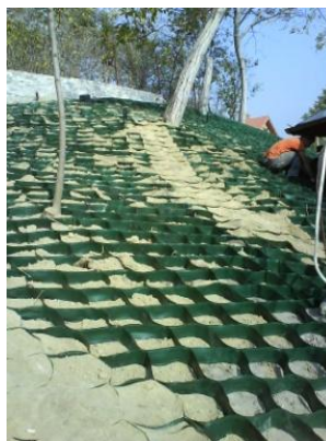
Fig. 9 – Filling the geocell with soil
