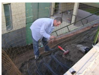
Fig. 4 – Installing armed layers with Buzau Mesh
