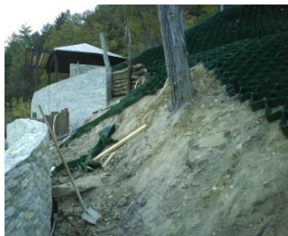
Fig. 11 – Joining the geocell strips
