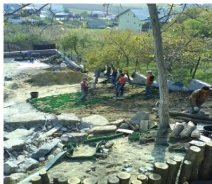
Fig. 12 – Midway stage of filling the geocells with soil
