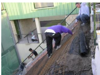
Fig. 5 – Fixing the arming
