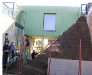
Fig. 6 – Fixing the armed embankment
