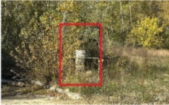
Figure 6 Pier with visibility blocked by vegetation on berm 2 of the downstream slope of the earth dam (photo author, 2025).
