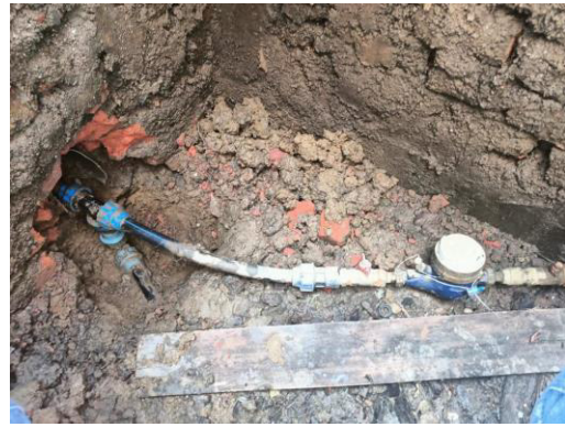
Figure 3 Illegal connection made upstream of the flow meter
