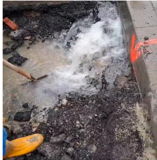
Figure 6 Detail of water loss at the branch
