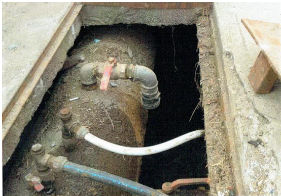
Figure 2 Illegal connections on the main water transport pipe
