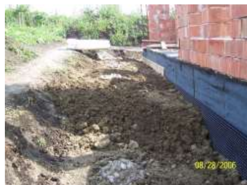
Figure 4 Drainage with filtering prism in constructions
