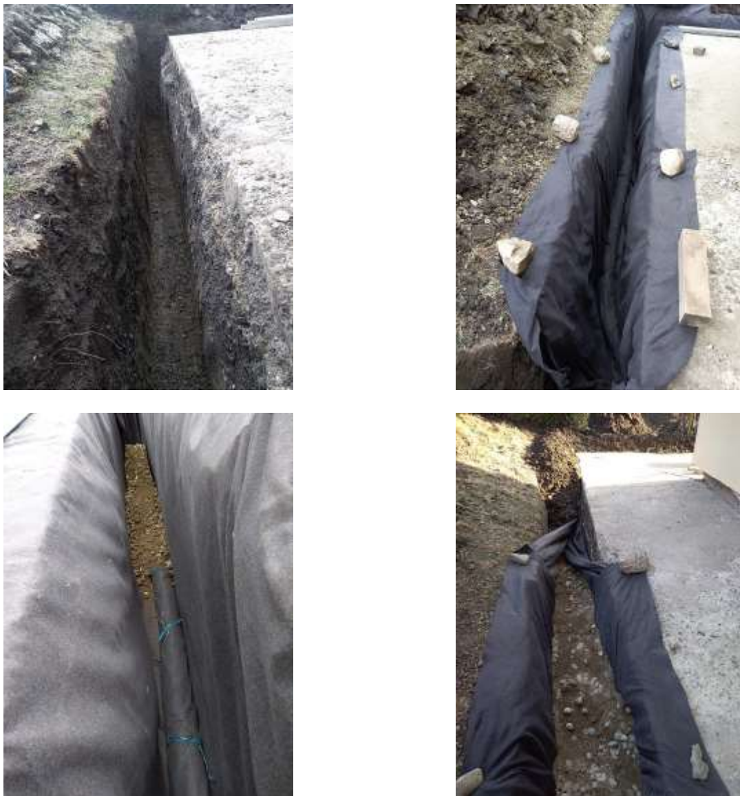
Figure 5 Doubling the marginal drainage
