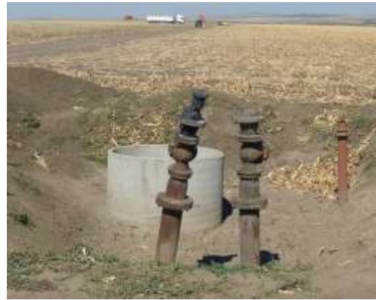
Figure 2 Degradation state of buildings and installations on the pipeline network of the plot Irrigation SPP1b (Luca, 2015)
