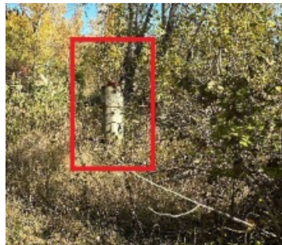
Figure 5 Pillar with visibility blocked by vegetation on the downstream slope of the earth dam (author photo, 2025).
