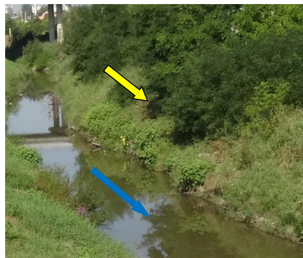
Figure 8 General view of the left bank at the minor bed of the Bahlui River on the research section (Luca M., 2019)
