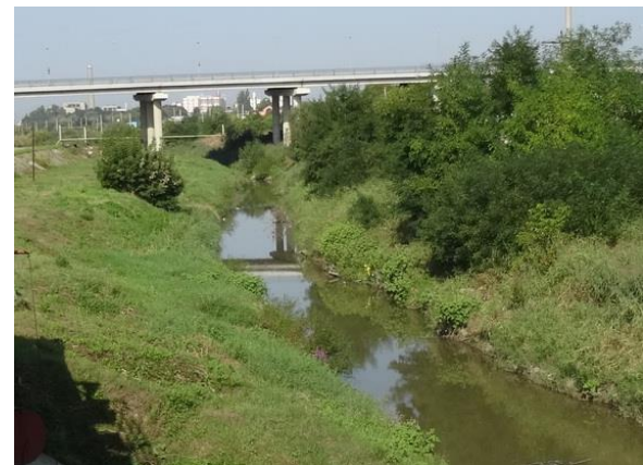
Figure 7 General view of the regularized minor bed on the research section (Luca M., 2019)
