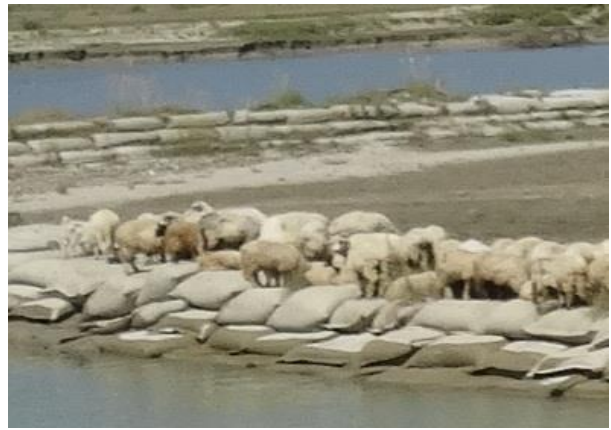
Figure 13 Degradation of the geo-bags located at the top of the coastal defence by the movement of sheep flocks (photo author, 2020)
