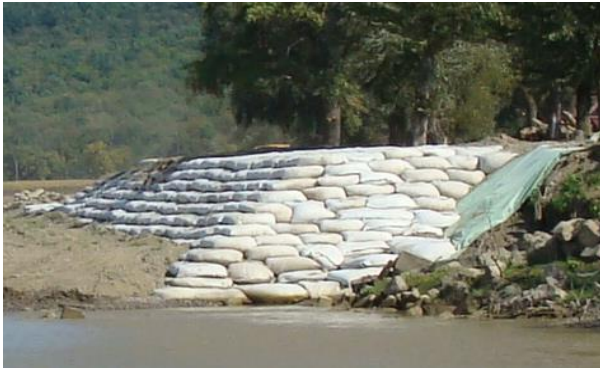
Figure 7 Execution stage of the shore defense with geo-bags on the Moldova river (photo Luca M., 2015)
