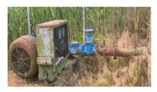
Figure 3 View of 7/5-2 pumping unit (6NDS), electric panel and discharge pipe of the SPPM 7/5 (Photo Luca M., 2016)
