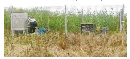
Figure 5 General view of Doniceasa-Fălciu Plot 7 SPPM SP 7/2, partially rehabilitated (replacement of electric motor and electric panel) (photo Luca M., 2016)
