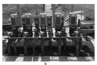
Figure 4 The pumping station SPP1b rehabilitated: a - general view; b - hydraulic installation.
