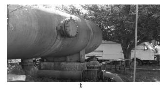
Figure 2 Details on the status of the pumping station SPP1b components: a - taps and check valves on the discharge line; b - hydrophor installation.
