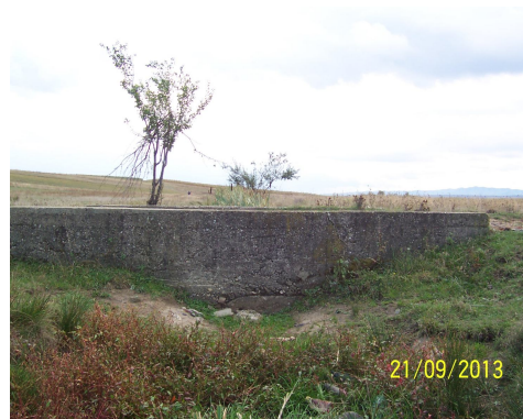
Figure 2 Blocked culvert
