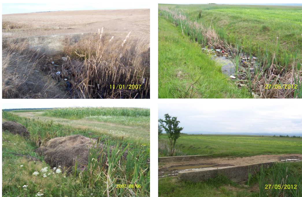
Figure 2 Clogged culvert showing vegetal and household residue within the canals
