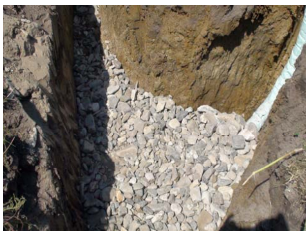
Figure 10 Connection of absorbing drainages
