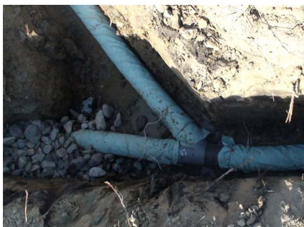
Figure 10 Connection of absorbing drainages
