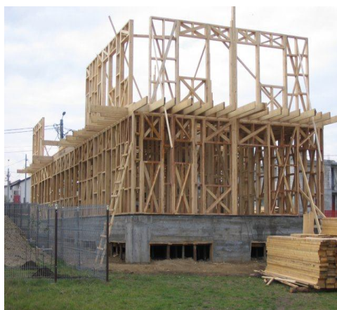
Figure 2 Foundation and structure of ecological wooden houses
