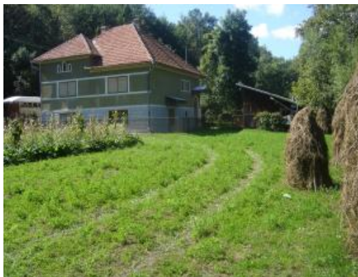
Figure 2. The old renovated building
